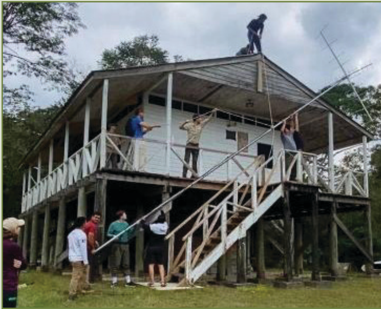
Motus tower being installed with the help of University of South Wales in March 2026.
